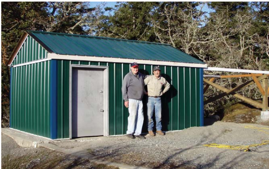
The roof is on - Geoff Jones and Bruno Quenneville - Happy volunteers
