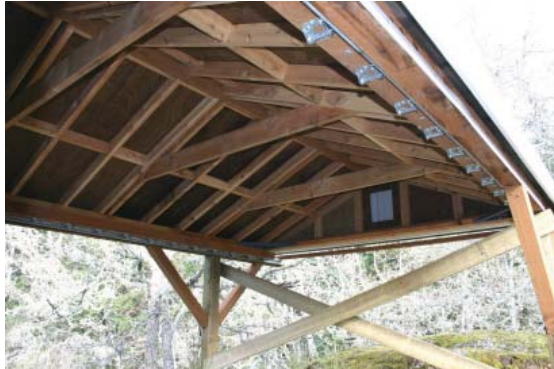
Inside view of extended roof
